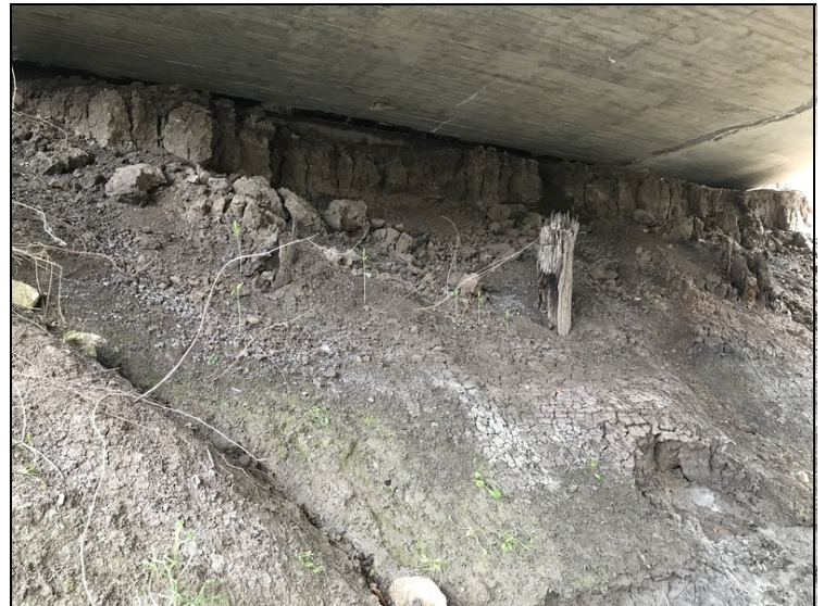
Abutment #2 slope erosion
