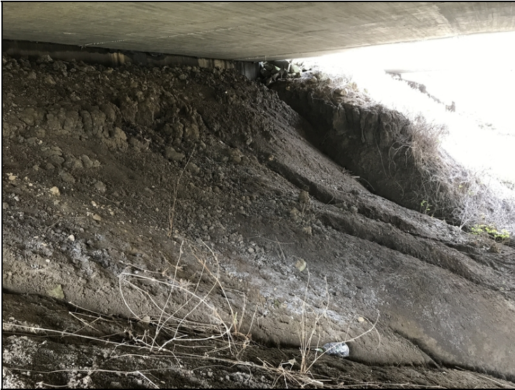
Abutment #1 slope erosion.
